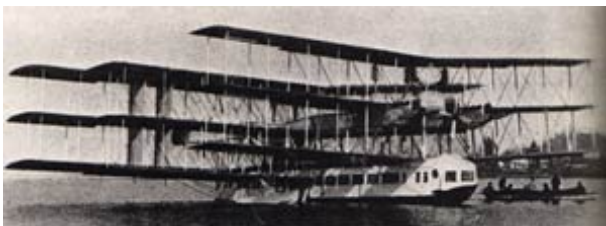
The Capronissimo, a nine wing seaplane, able to transport 100 passengers, 1921
