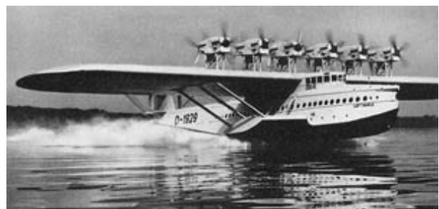
The Dornier DO-X, a 12 engine seaplane, able to transport 169 passengers, 1929
