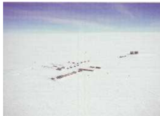
Fig. 1 An overview of the Dome C summer camp.
