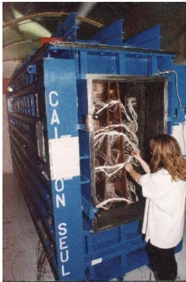
FIG. 3.54 – Temporary cabling of one sector in the special container before tests of the wire chamber.
