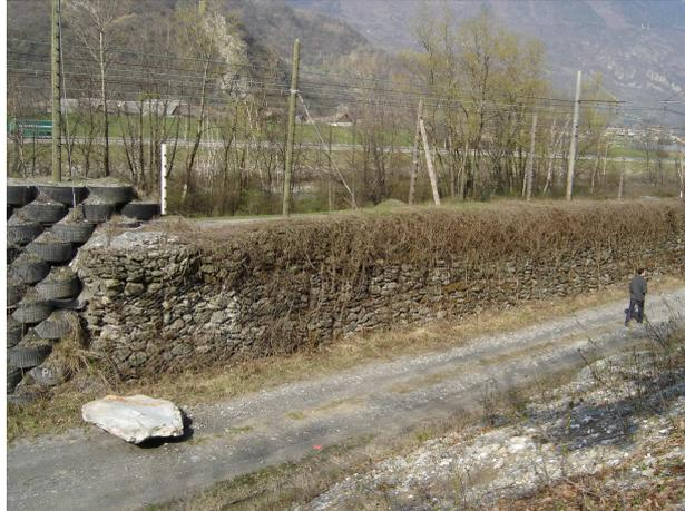
FIG. 1.7 – Merlon de protection construit en gabions (Photo Cemagref).
