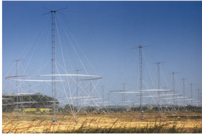
Figure 2.2: Biconical antenna of the HF skywave radar Nostradamus
