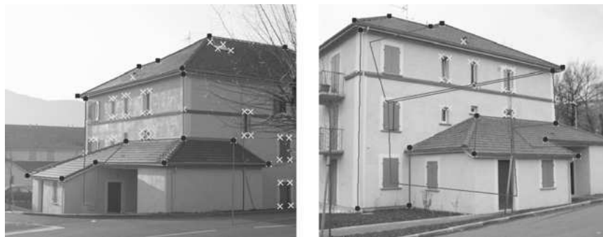
Figure 5. Reprojection of the recovered model onto the original images. The yellow crosses indicate the position of the reprojected point features.
