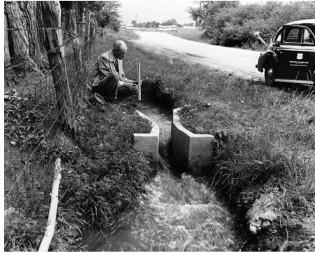
FIG. 1.2: Ralph Parshall, et son célèbre Parshall Flume (Copyright © 1946 CSU/Photography and Digital Imaging).
