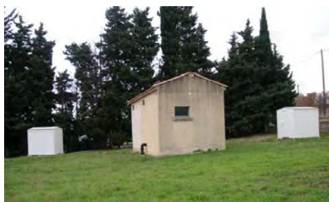
Figure 126. Captage de Paulhan (C12).
