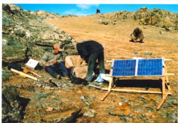
Figure IV.13 Images from the installation of the temporary network. The CMG40 sensor is installed on a concrete base. Two solar panels provide the alimentation.
