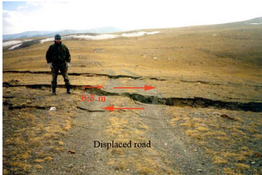
Figure III.8: Photo of surface rupture (for location, see Fig III.6). Road displaced with a right lateral strike slip. The displacement is 0.5 m on the first segment. If we add all segments, the total horizontal displacement is about 1.5 m.
