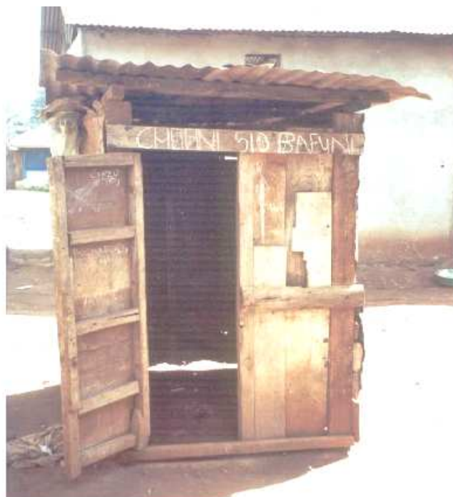
Latrines bas standing
