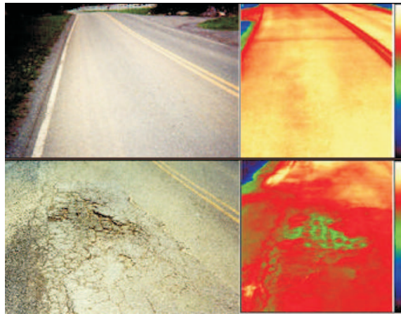
Figure 1.4: Road condition assessment using thermography.
