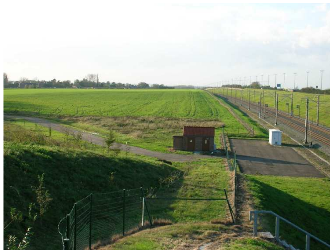
Figure E.1: Site of Lincet: overview of the measurement site (picture taken on November 3, 2005).
