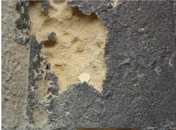
**Figure I-3.** Granular disintegration on St Etienne church, Fécamp, Seine-Maritime, France (limestone). This church is located 300m of the sea.
