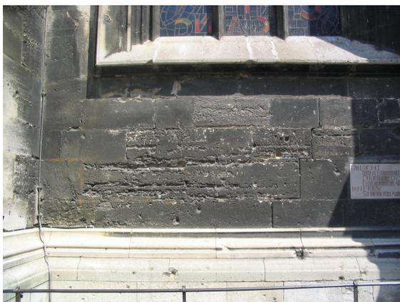
**Figure I-16.** Anisotropic weathering along the bedding on Stefansdom, Vienna, Austria (sandstones).
