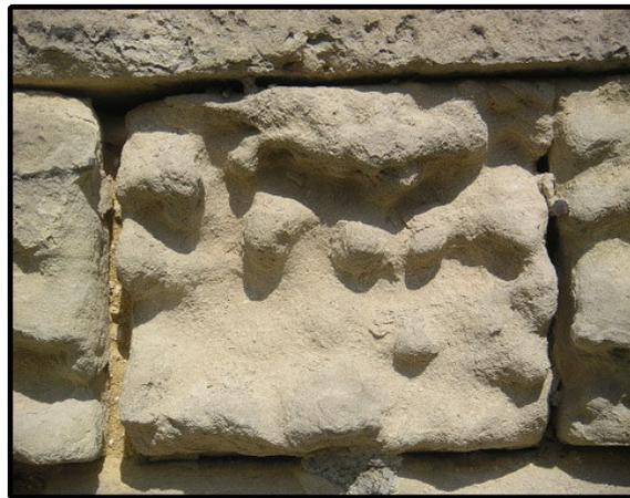
**Figure I-22.** Disjoining around the alveolated stone due to a high strength contrast between the limestone and the lime mortar. The size of the block is 40 cm. Cormeilles-en-Vexin church, Val d'Oise, France.
