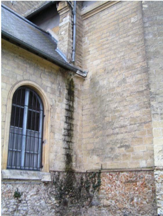
**Figure I-11.** Biological colonisation under a leaking gutter of the Neuville-sur-Oise church, Val d'Oise, France (limestone).
