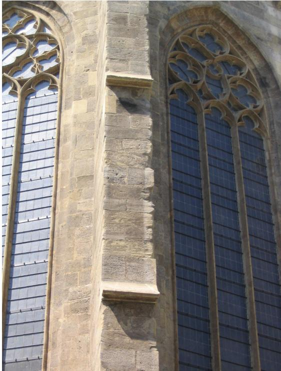
**Figure I-23.** Differential weathering of a buttress from the Stefansdom in Vienna Austria (sandstones). We can clearly notice that the right-hand part of the buttress is much more weathered than the left-hand part. This is certainly due to its orientation regarding the main wind direction.
