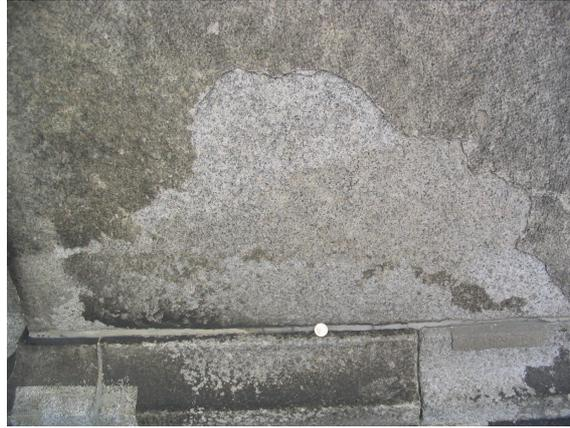
**Figure I-28.** Desquamation in granite due to the cement mortar used to repair the wall. Berliner Dom, Germany.
