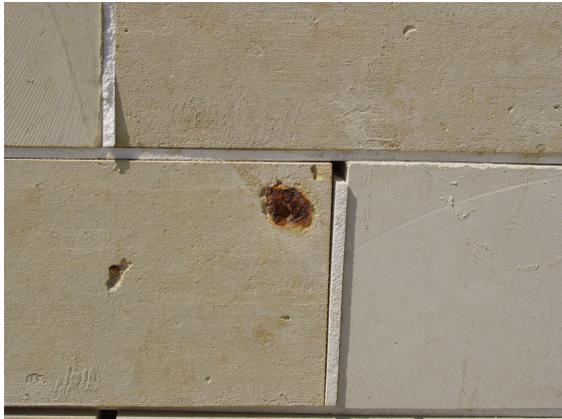
**Figure I-14.** Weathering due to a few centimetres pyrite inclusion in a very fragile stone, StCyr en Bourg, Maine-et-Loire, France (tuffeau).
