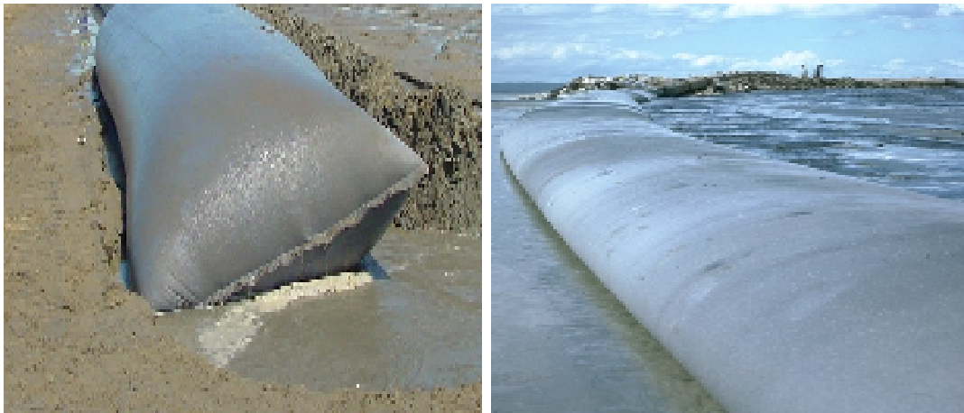
FIG. 4.4 – A geotextile tube before submersion. This LCS is a long cylinder made of synthetic textile and filled up with sand.
