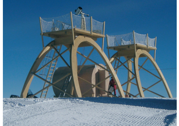
Fig. 1. Concordiastro observatory in November 2004. One can see the two platforms and the wooden igloo between. The DIMM is on the top of one platform.
