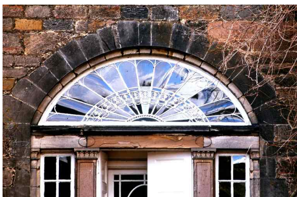
Figure 3.34 A window of Seton Castle, Scotland illustrating the need for controlling stone arrangements.
