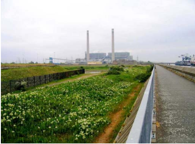
TILBURY POWER STATION and TIDAL WALL
