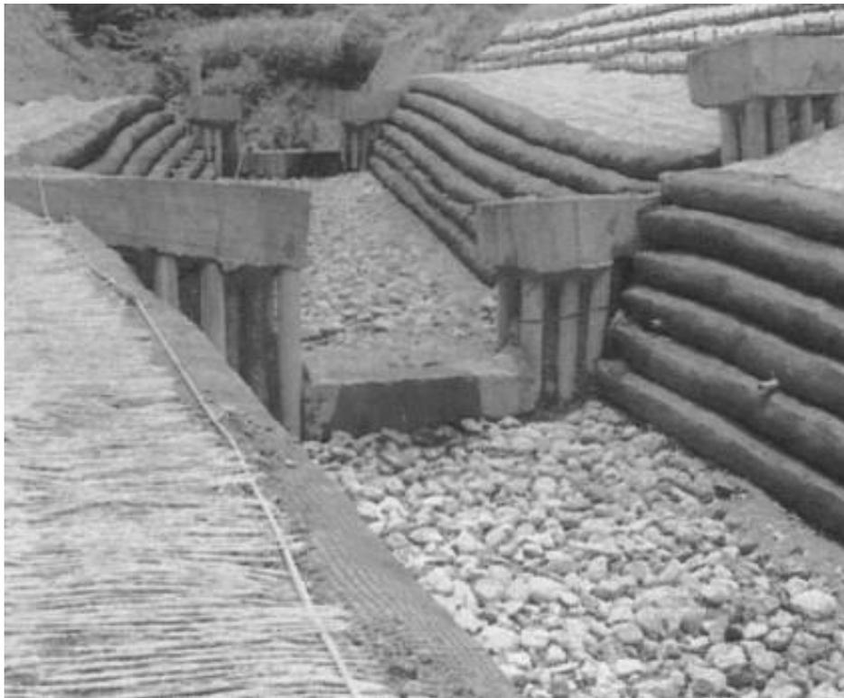
Figure 3.9 The reinforced revetment using geotextile.
