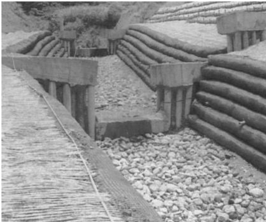
Figure 3.9 The reinforced revetment using geotextile.
