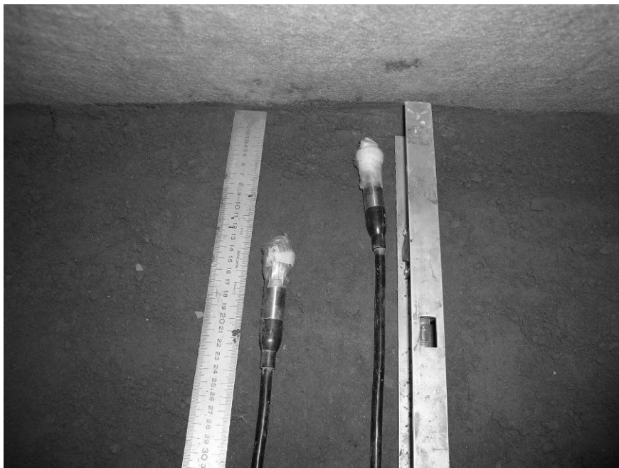
Figure 3.5 Water pressure monitor - piezometers.
