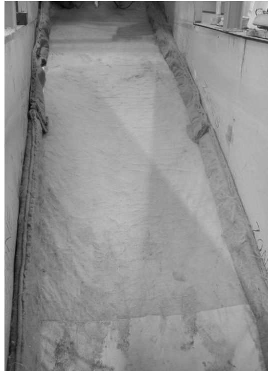
(b) Laid the geotextile and geotube.
