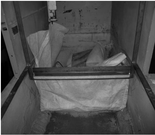
(a) Fix the geotextile bag on rack.
