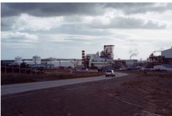
68.Installations Cabo Negro
