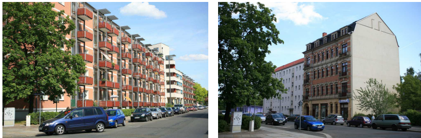
Figure 5.51: Optical image. Left: Building number two, right: Building number three (copyright G.S.).
