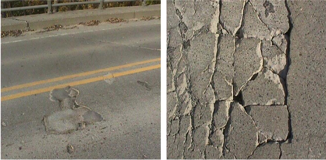
Figure 1.3 Examples of extensive cracking and potholes in concrete bridge deck
