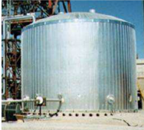
Figure 4.12 – Cuve de stockage [170]
