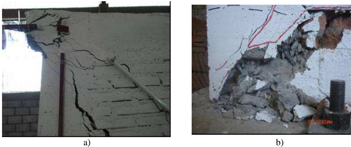
Figure 4.30: a) Compression failure at the load application zone, b) Flexural failure of the longitudinal reinforcement and shear failure of the concrete section
