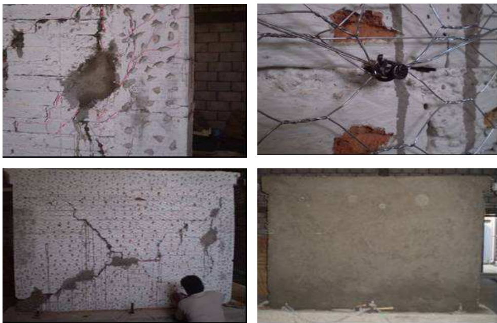
Figure 4.34: Retrofit process of the wall MMR2
