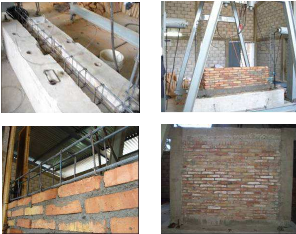
Figure 4.22: Construction process of confined masonry walls
