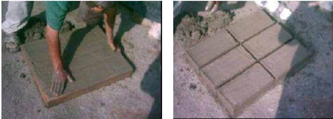
Figure 2.3: Manual process to obtain solid clay bricks
