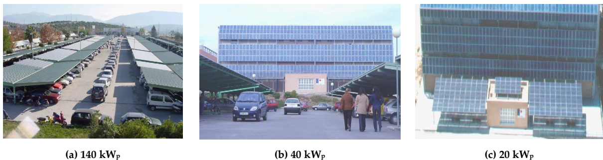
Figure III.11 : Views of (a) solar parking 1 & 2 PV arrays, (b) facade PV installation, and (c) pergola installation [PER'07]
