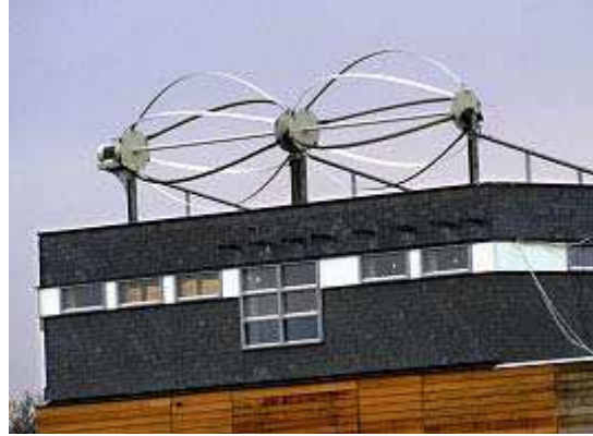
Figure I 12 : Source : Eolienne de type Darrieus (WindWall)
