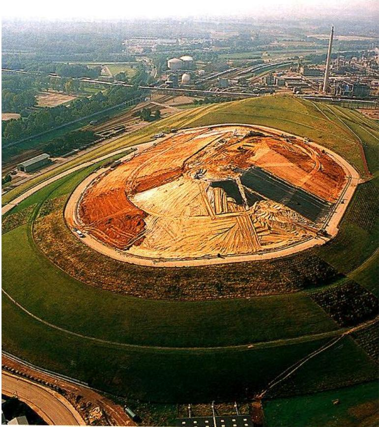
**Figure I-10 : Construction of landfill cell according to area method (French landfill site).**
