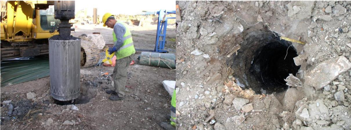
**Figure VI- 42: Waste extraction at landfill site ‘N’.**
