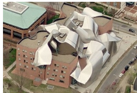
Fig. 5-8: Weatherhead School of Management – Cleveland – USA – Gehry & Partners – 1997 / 2000
