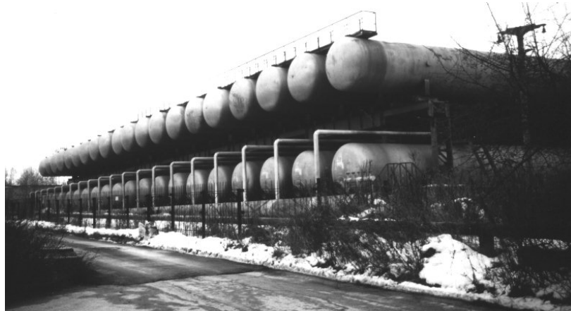
Figure 4.2: Air storage for T-313, up to 20 bar.
