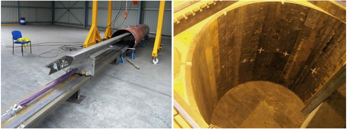
Figure 5.15: Left plot: Demagnetization process of the shielding bars. The V shape of the bar can be viewed. Right plot: shielding integration during the summer 2008.
