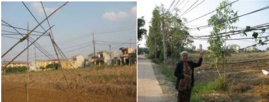
Figure 1-15: The electricity distribution systems exist in rural areas.
