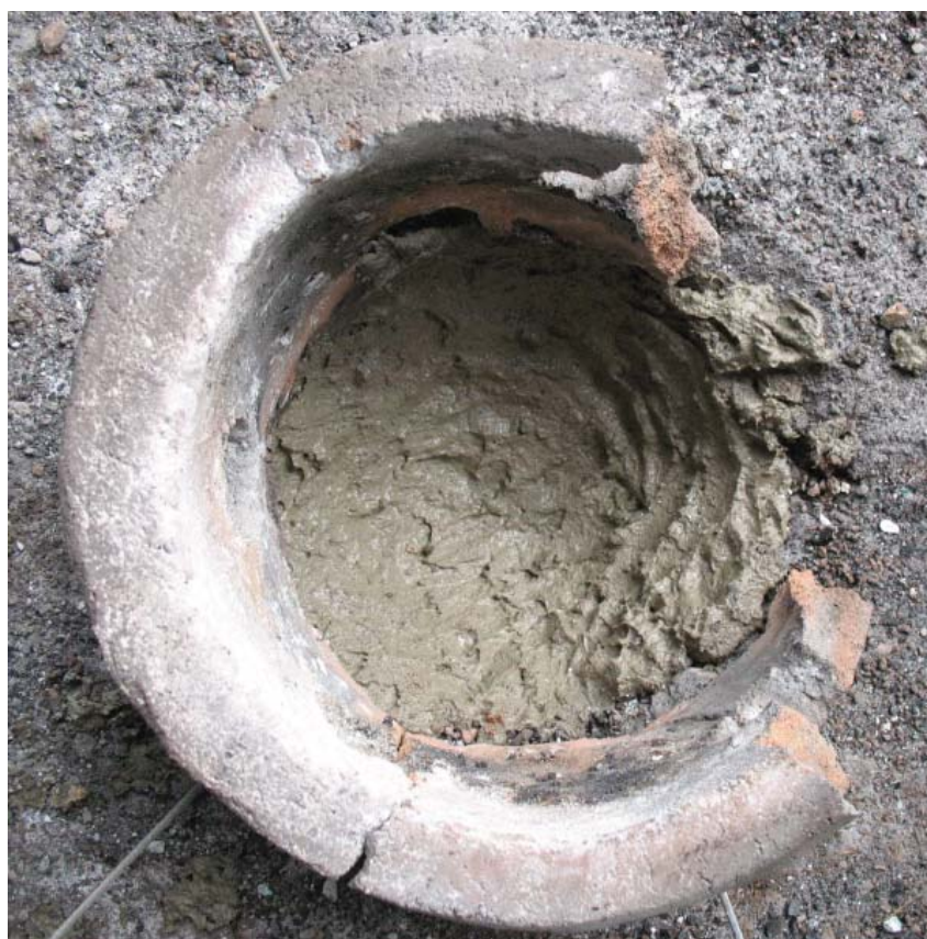
Figure 7.21 - Furnace chimney from Burn 5 being repaired for Burn 6, and placed over a clay-lined pit. Image: author.
