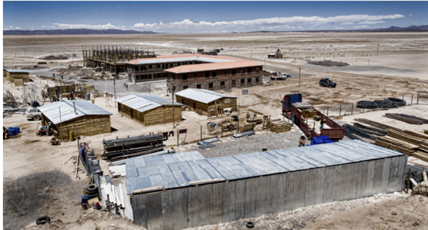
Figure 3.5 – Pilot lithium plant under construction in Uyuni [99]
