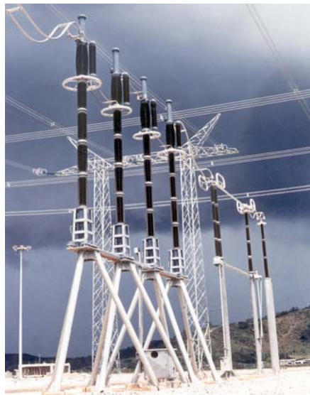
Fig. 3-19 : FX42D circuit breakers
