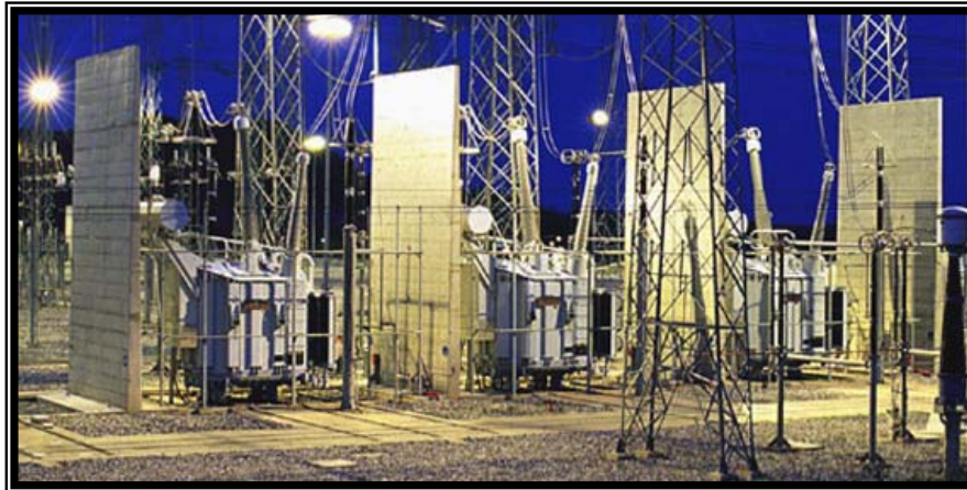
Fig. 3-48 : Illustration of firewalls for power transformers
