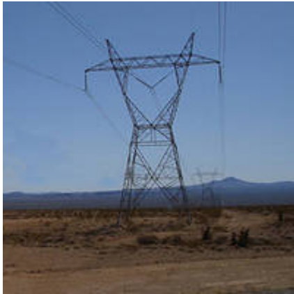
Fig. 3-9 : IVI insulator strings
