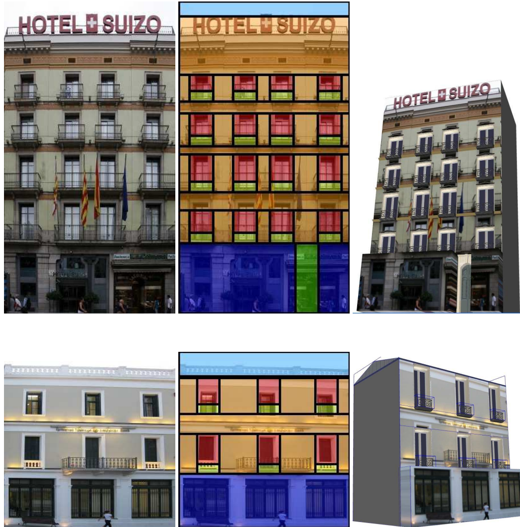
Figure 4.16: The method is still able to cope with even more different architectural styles, such as Barcelona architecture (first row), or Greek Neoclassic buildings in Heraklio, Greece (second row).
