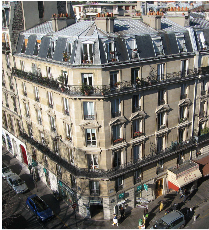
Figure 3.16: A typical building from the early Haussmannian period.
