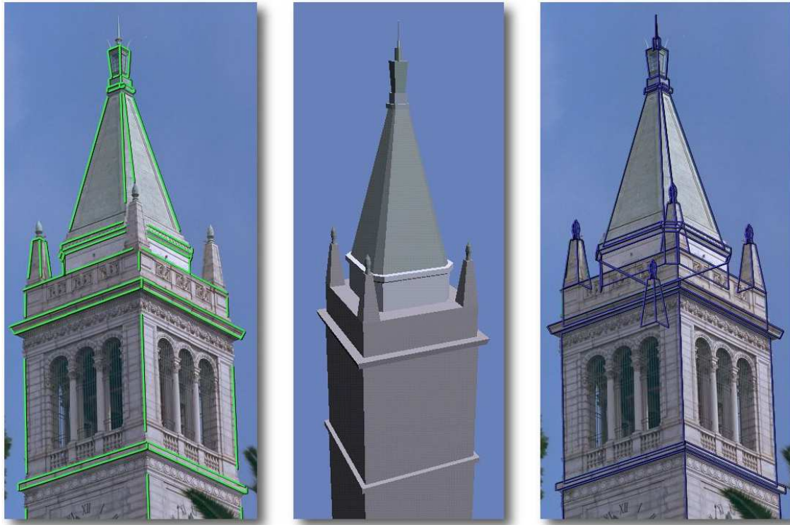
Figure 2.5: Because of their high repetition rate in architecture, some common configurations of planes should be taken as primitives by themselves. The example (a photograph of the Campanile, Berkeley's clock tower) shows many instances of prisms and parallelepipeds. Image courtesy of [Debevec 1996].
