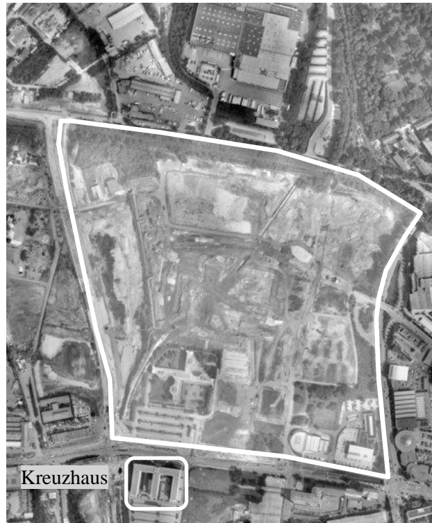
Figure 2.1: The main excavation area Site
