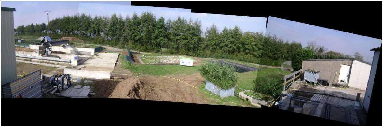
Figure 7. Construction of the system; view from the piggery.
