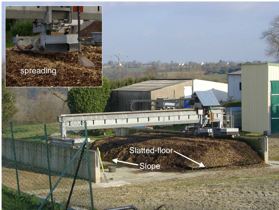
Figure 10. Vermifilter (width: 4m, length: 10m, height: 0,6m)
