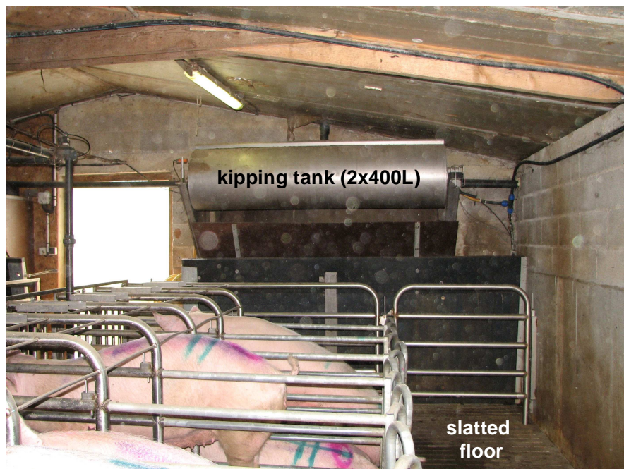
Figure 8. Kipping tanks used in the piggery for effluent flushing
