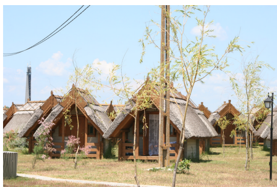
Fig. 2.6 Bungalows del camping "The Dolphin"
