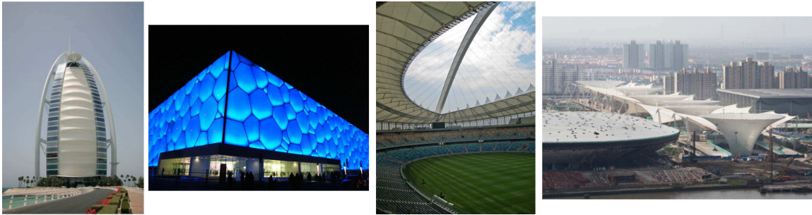
Figure 1.2: From left to right: Burj Al Arab Hotel in Dubai (with a textile façade); the Beijing's Water Cube; the Moses Mabhida stadium in Durban, South Africa; and the 2km length textile-covered entrance to the EXPO in Shanghai 2010
