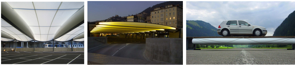
Figure 1.3: Sample Tensairity ® applications. Left and center: parking cover (sources: canobbio.com and tensinet.com); Right: deployable bridge (Source: Buildair)
