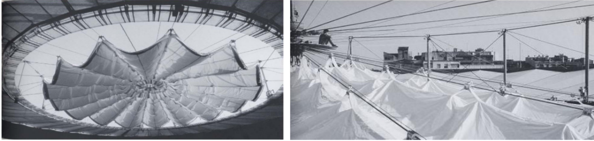
Fig. 2.47: The retractable part of the Bullfighting Arena roof in Zaragoza (architect: J. Schlaich) [Sobek, 1999] (cited by [Walter])
