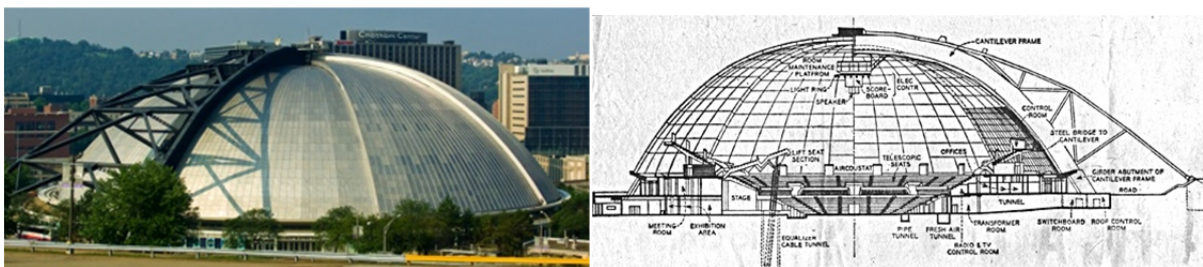
Fig. 2.5: Pittsburgh Civic Arena (architect: Mitchell and Ritchey) photo [Lorentz, 2008] and original blueprint [Helvenstone, 1959]
