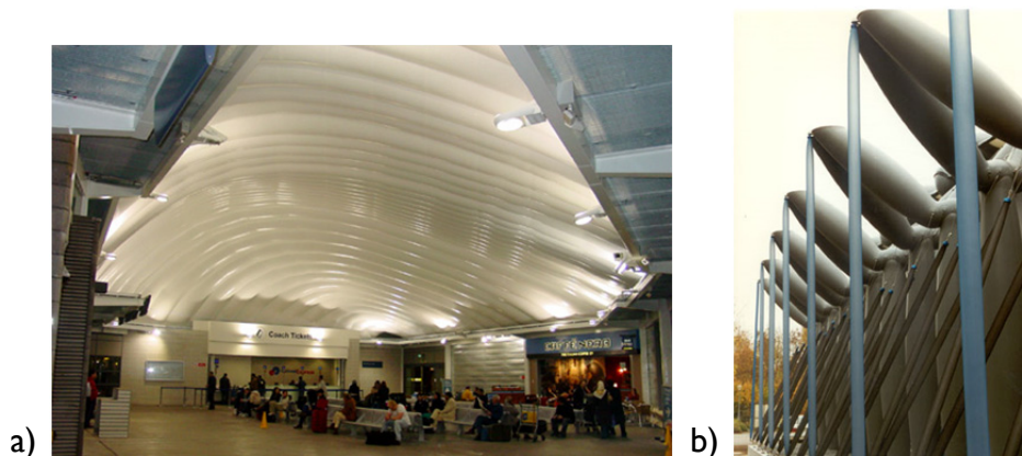
Fig. 2.50: a) Inflatable roof for Heathrow airport central bus station (architect: D5) [Lindstrand, 2006]; b) 19.5 m x 40 m Exhibition Hall with air-inflated elements (architect: Festo AG & Co) in Germany [Festo]
