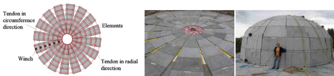
Fig. 2.53: Transformation of precast divided planar segments into a hemispherical dome [Dallinger and Kolleger, 2009]
