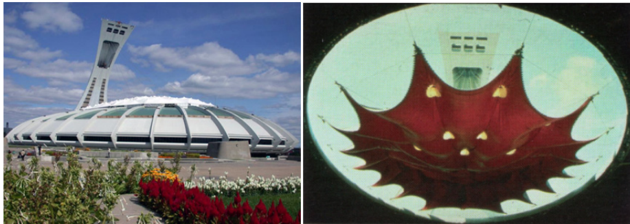
Fig. 2.46: Olympic Stadium in Montreal (architect: Roger Taillibert) [Tolivero] and its original retractable membrane roof [Barnes, 2000]
