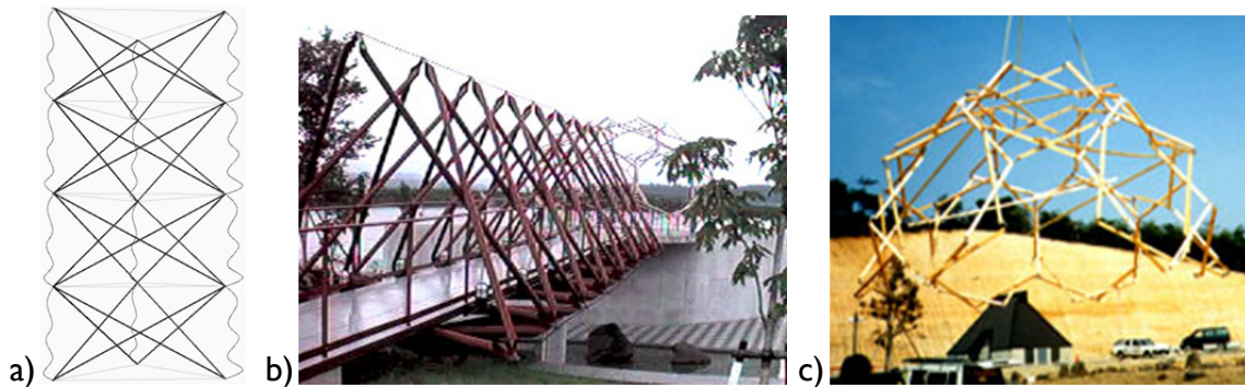
Fig. 2.21: a) Deployable mast controlled by active and passive cables by the former Deployable Structures Laboratory; b) foldable bridge and c) deployable dome by ATAKE Space Design Lab. Co. in the Hanamizuki Park, Japan [Atake]
