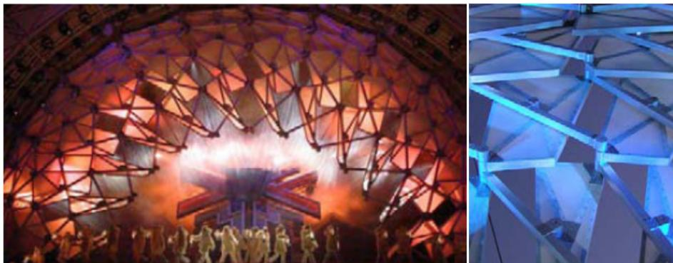
**Fig. 2.32:** Cover solutions for retractable structures by Hoberman: transforming Olympic Arch for the 2002 Winter Olympics (Salt Lake City, USA) designed by Hoberman [Hoberman]
