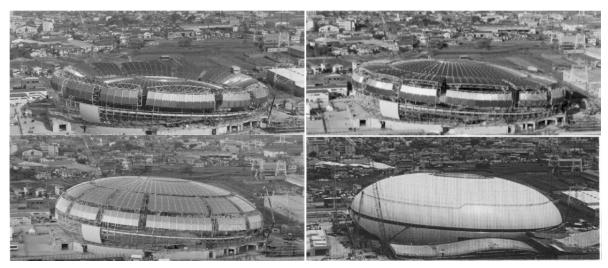
Fig. 2.34: Erection of Namihaya Dome (Showa Sekkei Corp), Osaka, 1997 [Kawaguchi, 2002]
