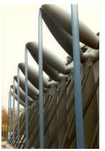
**Fig. 2.50:** a) Inflatable roof for Heathrow airport central bus station (architect: D5) [Lindstrand, 2006]; b) 19.5 m x 40 m Exhibition Hall with air-inflated elements (architect: Festo AG & Co) in Germany [Festo]
