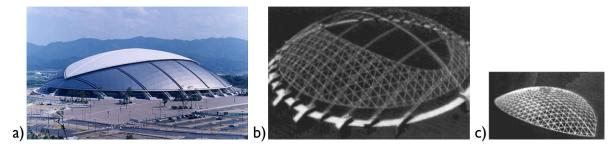
**Fig. 2.8:** Oita Stadium (architect: Kisho Kurokawa) a) photo [Ezinemark, 2010]; b) fix structural part [Ishii, 2000] and c) retractable top section [Ishii, 2000]
