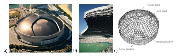
**Fig. 2.6:** Fukuoka stadium (architect: Takenaka Corp.) a) photo with closed [Yahoo, 2010] and b) with opened roof (Japan Atlas) c) structure [Ishii, 2000]
