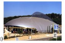
**Fig. 2.51:** a) Inflation of formwork; b) shotcreteing on the inside of the membrane; c) irregular shape structure constructed with pneumatic formwork [Pirs SA.]
