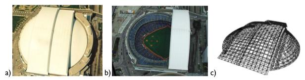
**Fig. 2.10:** Toronto Skydome (architect: Rod Robbie) a) photo of closed and b) opened roof c) the structure of the retractable roof [Ishii, 2000]
