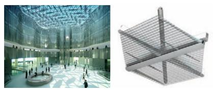
**Fig. 2.14:** Adaptive shading system of the Audencia Provincial, Madrid (by Hoberman and Fox+Partners) and the model of a hexagonal retractable panel [Hoberman]
