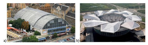
**Fig. 2.9:** a) Retractable roof of the Komjádi swimming pool [Komjádi]; b) Qi Zhong stadium (architect: Mitsuru Senda), [Ezinemark]
