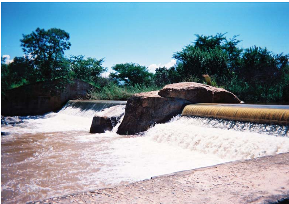
This picture was taken at the take-off weir. It needs special attention as it is silted but a lot of farmers depend on this place. (Participant n°32, New Forest B, 2009)
