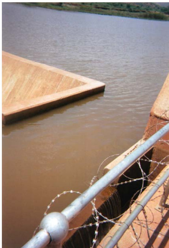
This is at the dam. The picture is showing the fence that is there to prevent children from getting in. I took this picture to show where the water we use come from.
