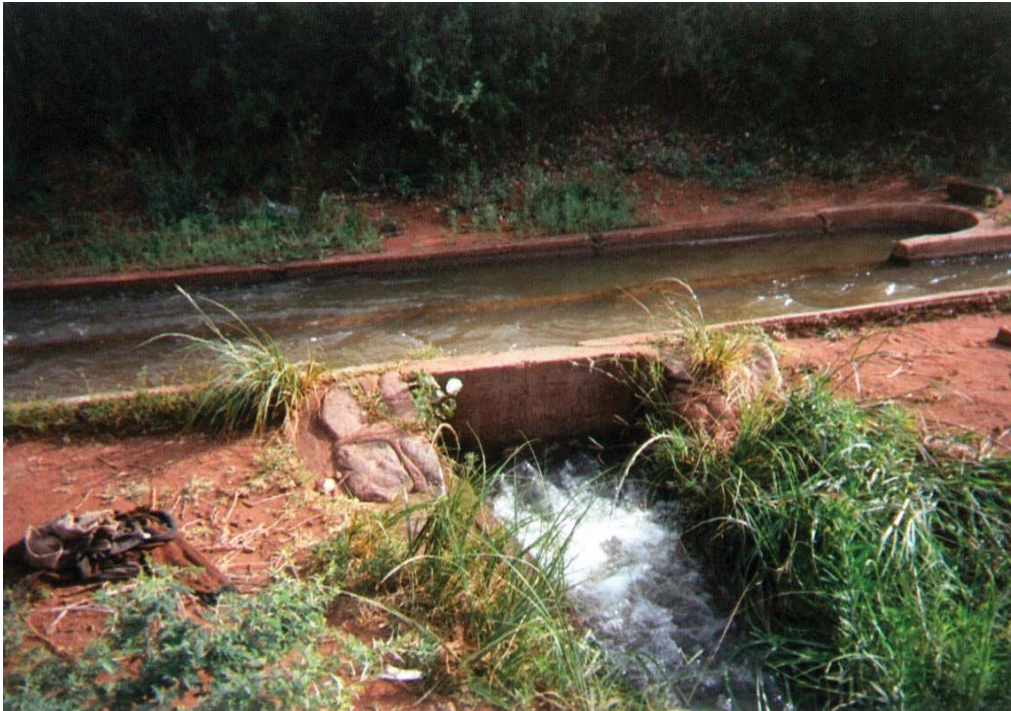
This is the main canal. The water comes from the dam. We open it to the secondary canal that we use to irrigate. (Participant-comité de Nzhelele n°10, Mphephu, 2008)
