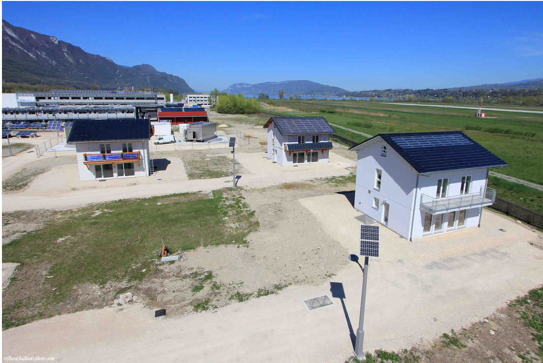
Figure 2.1 – Plateforme INCAS, INES, Le Bourget-du-Lac
