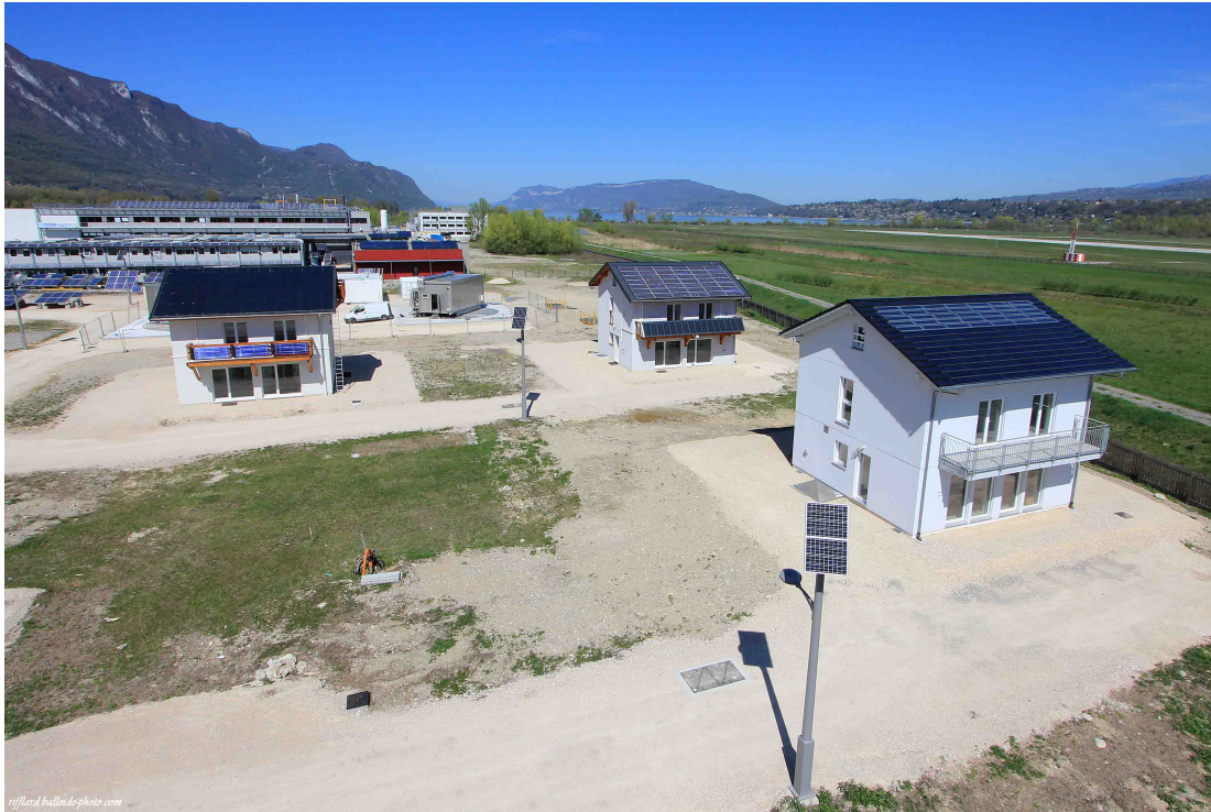
Figure 2.1 – Plateforme INCAS, INES, Le Bourget-du-Lac
