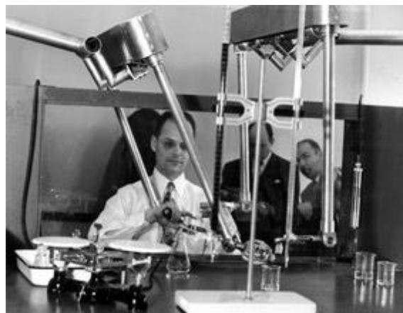
Fig. 2.9. The first teleoperation system developed by (Goertz 1952)
