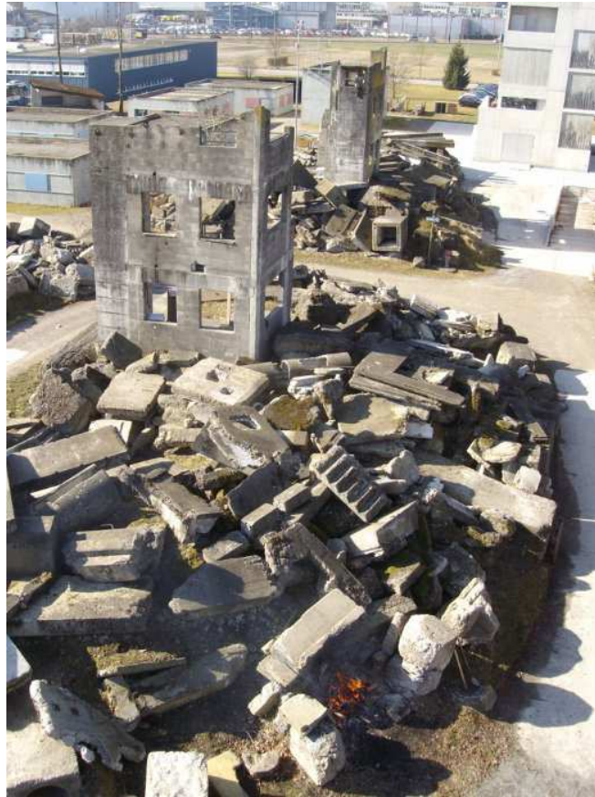
Figure 6.17: The firefighter training area in Zurich: the selected site for the final demo of the sFly project.
