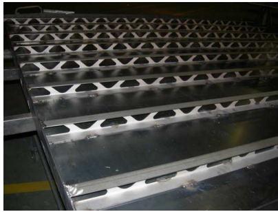
(a) Lower face with stiffeners.
