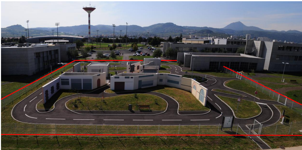
Figure III- 38 La plateforme PAVIN – Circuit urbain
